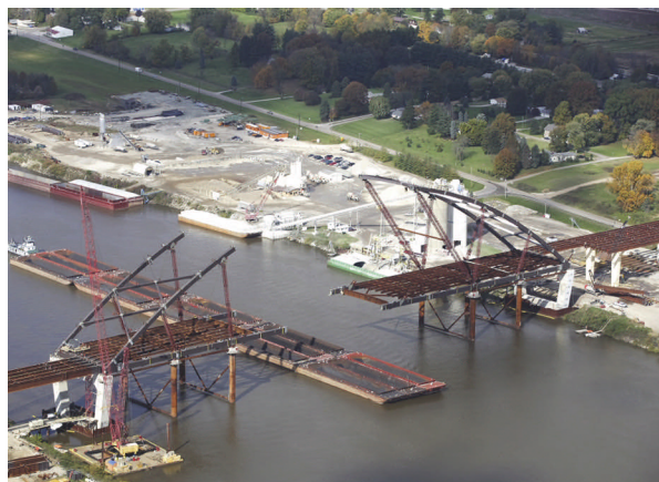
Constructing the networked, tied-arch span of the Blennerhassett Island Bridge over the Ohio River in 2007.
