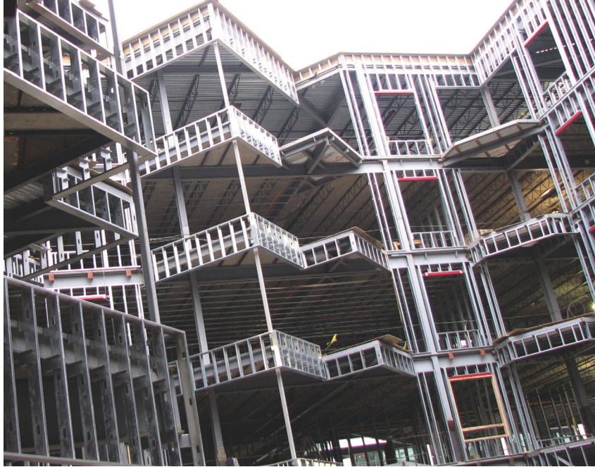
Thirteen vertical posts at the points of the plan projections support the third, fourth and fifth floors, reducing the number of weld-through beam connections required from 188 to just 26 on the second floor.
