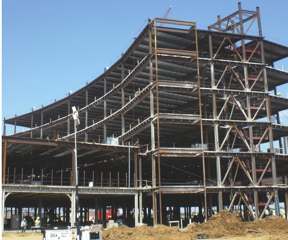
The architect's use of structural steel braced frames instead of concrete shear walls expedited the construction schedule.
