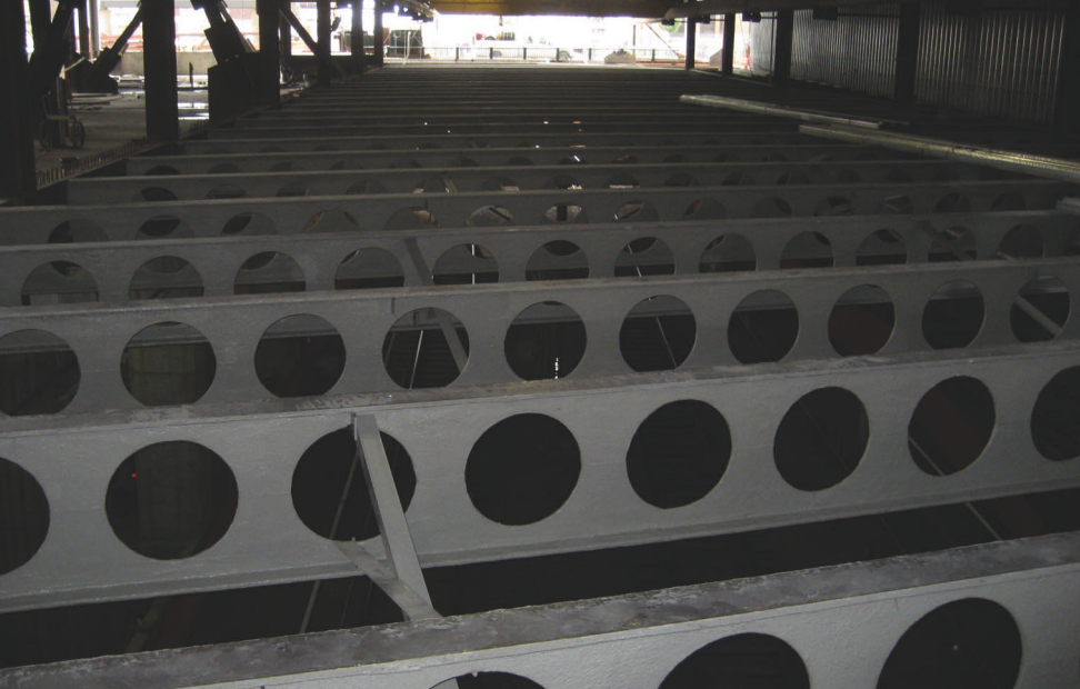
The St. Louis MetroLink rail lines are visible beneath the cellular beams for the base floor of the new BJC Institute of Health at Washington University, which all had to be placed between 1 a.m. and 3 a.m.
